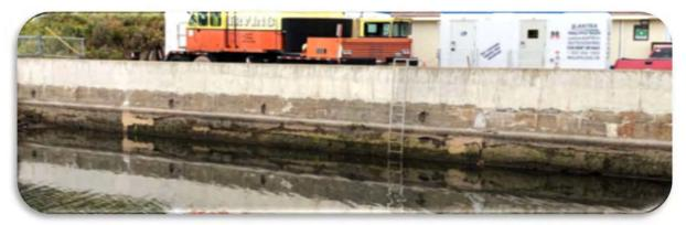
Photo 7: Photograph Showing the Deteriorating Condition of the Concrete Walls in the Forebay Area
