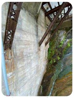
The structural inspection of the tailrace area indicated that repairs should be completed in the next five years (by approximately 2025) to reduce further structural damage. The
