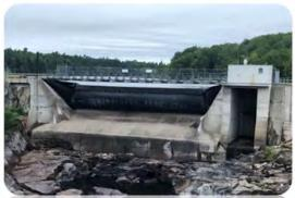
Photo 5: Sluiceway Bladder Sitting atop the Sluiceway, with the Spillway to the Right of the Photo underneath the Rubber Dam Control Building
