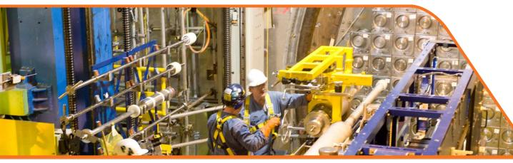
Workers at the Point Lepreau Generating Station install calandria tubes in the reactor vessel.
